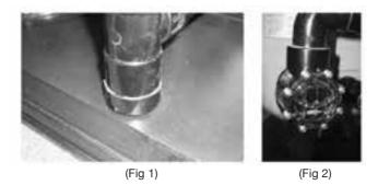
Regularly check the 3mm vent hole on the Blower pipe 'T' to ensure it is unobstructed allowing moisture to drain from the unit. (Fig 1)
