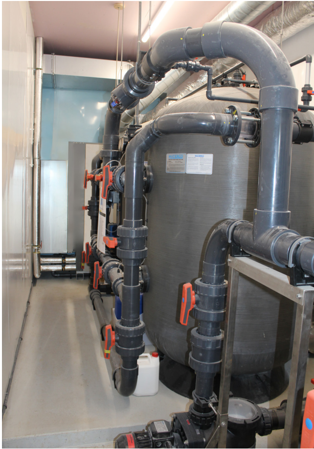
The heart of the plant room are installed 2 x SMDD1200 sand filters for the ultimate in filtration and water saving benefits.
