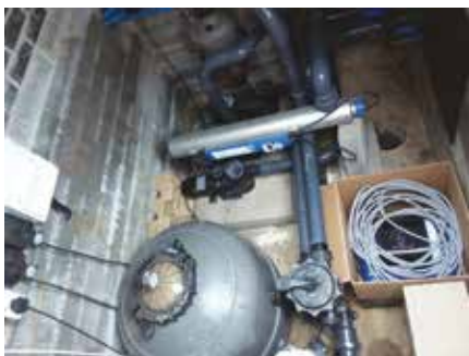
Waterco's Exotuf bead filter, Aquamite 1.25 pumps and a MultiCyclone MC16 with automated valve.
