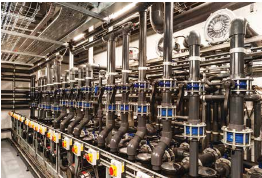
Waterco commercial pumps are corrosion resistant thermoplastic pumps, purpose built for commercial swimming pools.
