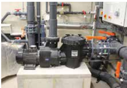
Hydrostar Plus pumps are high performance corrosion resistant thermoplastic pumps, purpose built for aquatic facilities, water parks and large commercial swimming pools.
