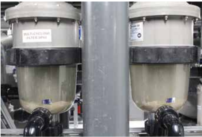
The addition of the multicyclones removes up to 80% of the incoming dirt through its multiple hydrocyclones prior to the water entering the main filtration system.
