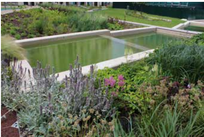
Cascading features designed to link the water play area with the main fountain pool.
