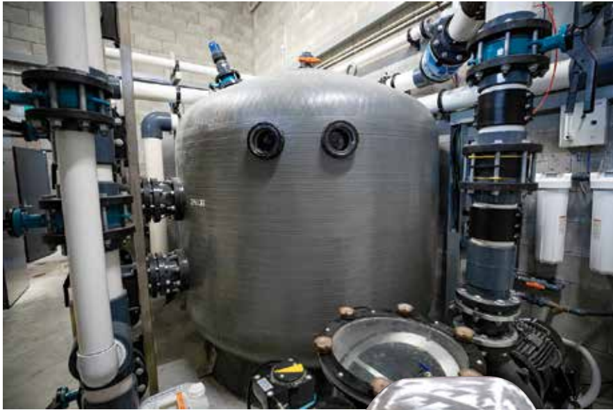
Waterco's revolutionary winding technology further strengthens the fiberglass filter tank, some models can withstand a working pressure of up to 1,000 kPa (150psi).
