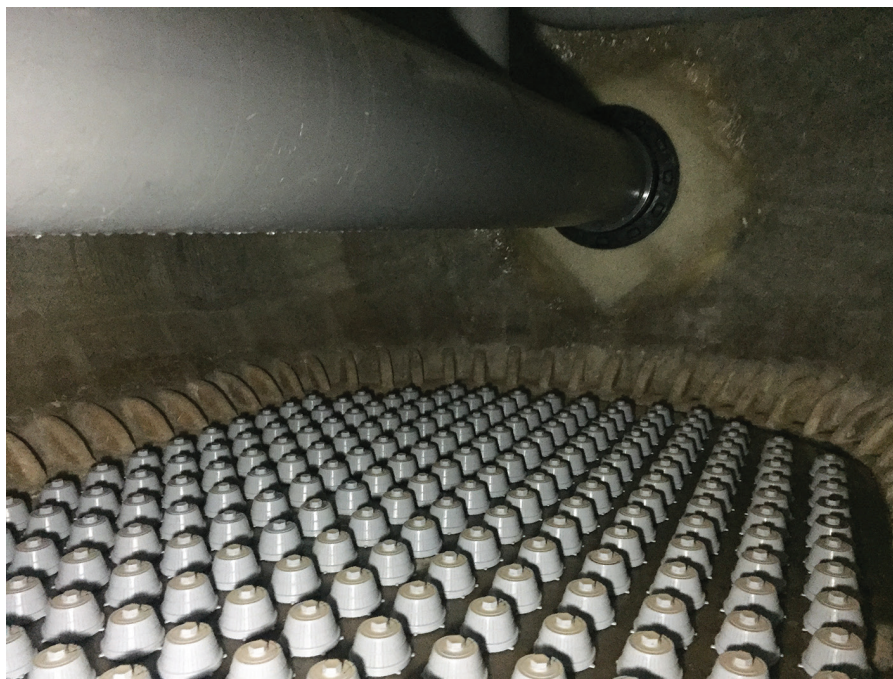
Nozzle plate filters are fitted with a plate and nozzle system, which ensures uniform flow for both filtering and backwashing. This provides maximum performance through the media bed.
