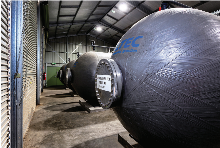
Fibreglass vessels have a mechanical and chemical resistance superior to steel, plus fibreglass does not rust or corrode and is able to withstand damage from many types of water treatment chemicals.
